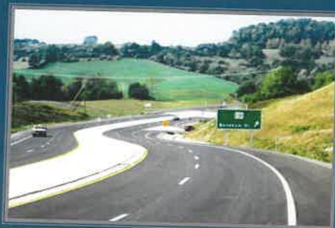
North Bridgeport Bypass
