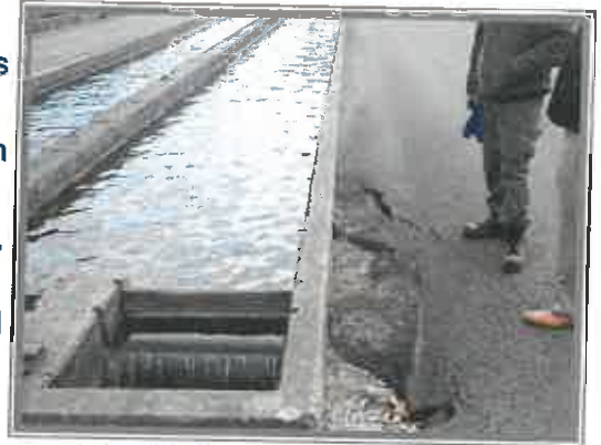
The site has space available for additional raceways.
